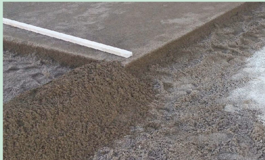
Laying G MIX
