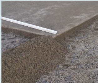
Laying G MIX
