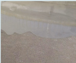
Laying GEOLEVEL self-levelling cement
