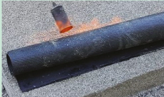
Bitumen sheet welding
