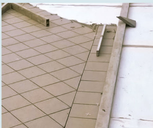
Application of tiles
