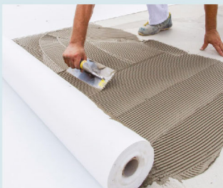
Application of GEODRY
